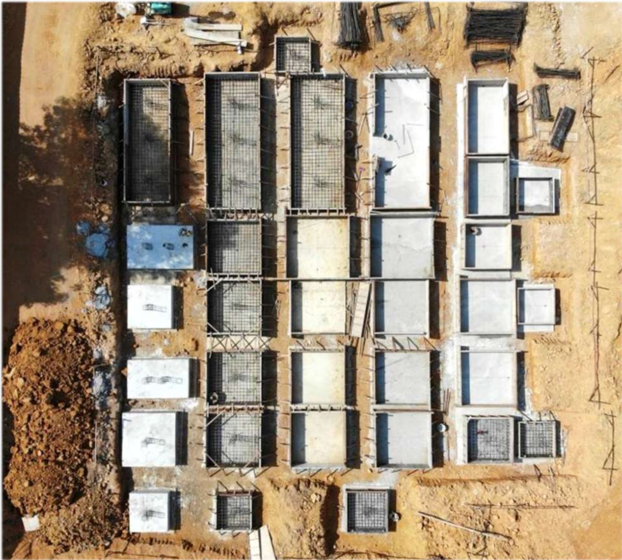
Figure 7 – Electrical Substation Foundations
