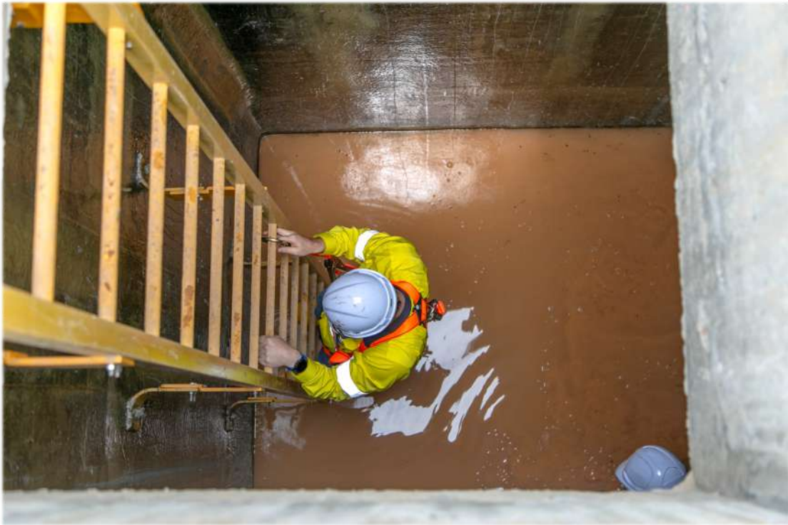
Figure 5 – Inspection of the OSD Tanks
