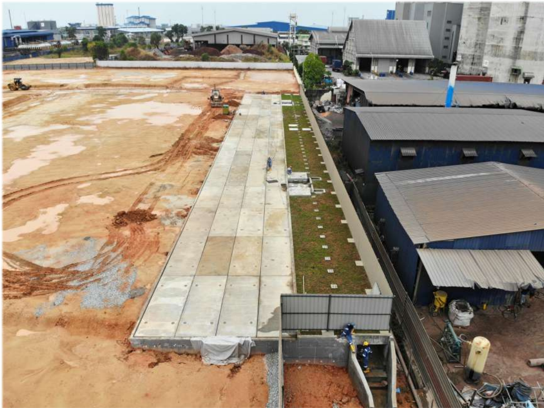
Figure 4 – Completed OSD Tanks
