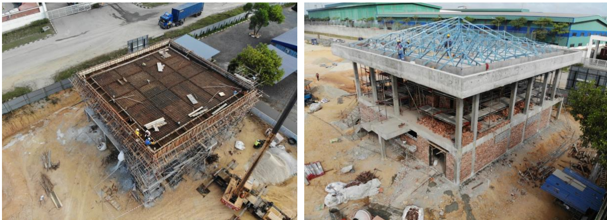
Figure 3 – Electrical substation roof construction, early January 2020
