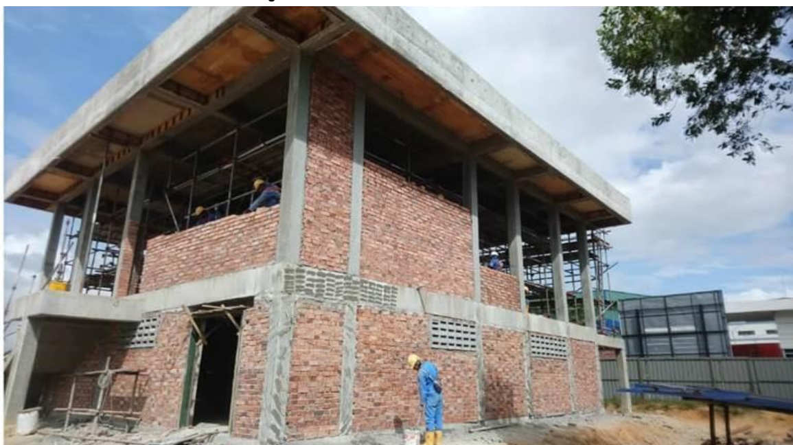
Figure 1 – Electrical substation construction
