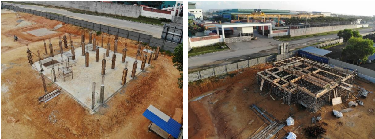
Figure 2 – Electrical substation initial works, December 2019
